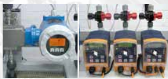
Use of high quality components: Magneto-inductive flow rate sensor and metering pumps
