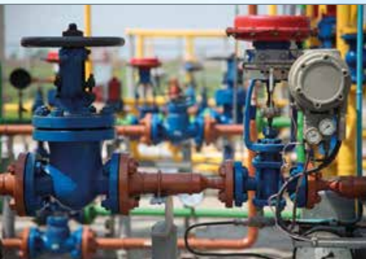
Redundant pumps: depending on the settings of the valves and fittings, either the right or the left pump is used.
